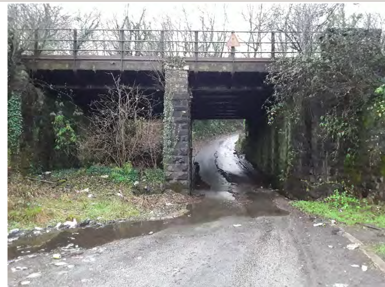
Plate 32: Railway bridge along cable route
