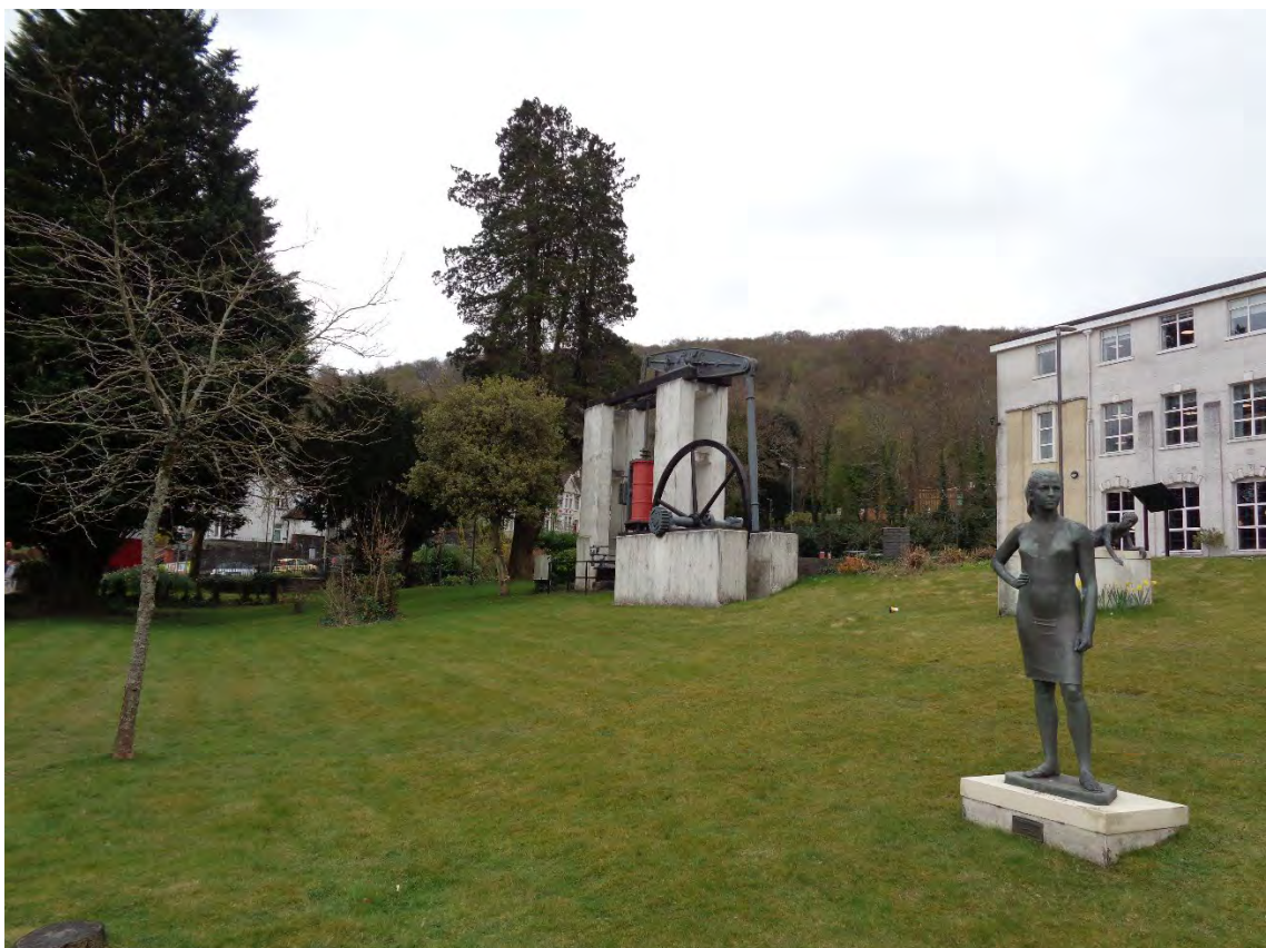
Plate 16: The Newbridge Beam Engine
